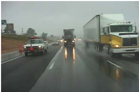
The photo above: I-35 in San Antonio, A-R on left and old concrete on right. The photo on the left shows an open surface in the far left lane where the water is not present at the tire pavement contact compared to a dense mix used in the rest of the lanes during a highway widening and resurfacing project.
